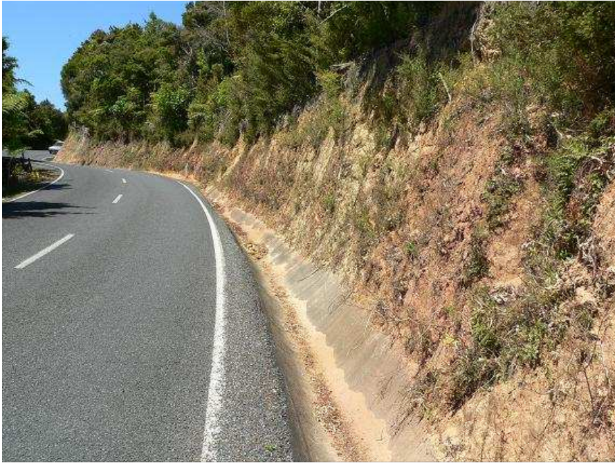
Figure 2.13 Large quantities of tumuli accumulating in the roadside drains on Mt. Tiger.
